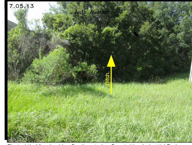
Photo 14) View Looking Southeasterly - County Line Industrial Park
