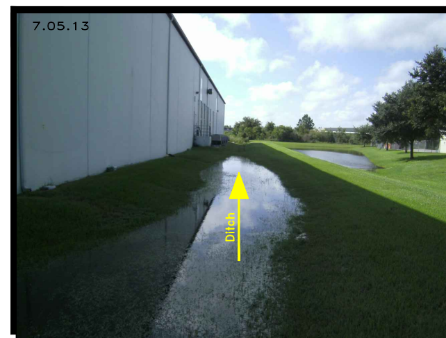
Photo 15) View Looking Southeasterly - West Lakeland Business Park
